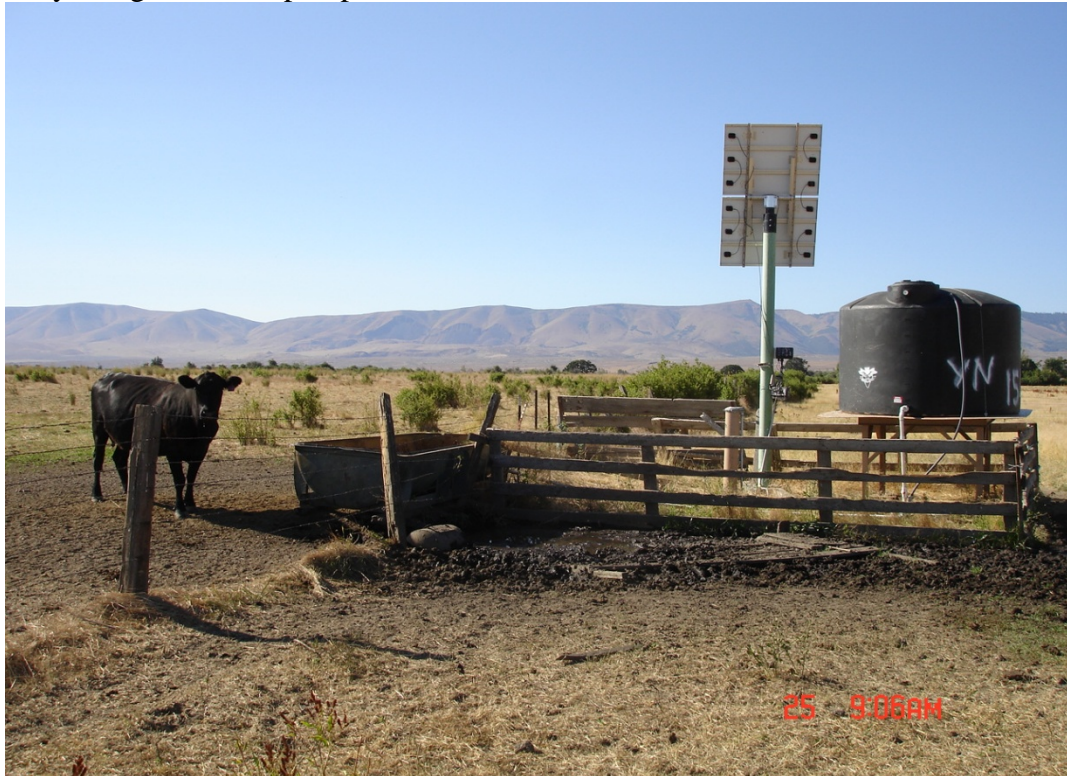
Figure 18. Stock pump and watering trough.
