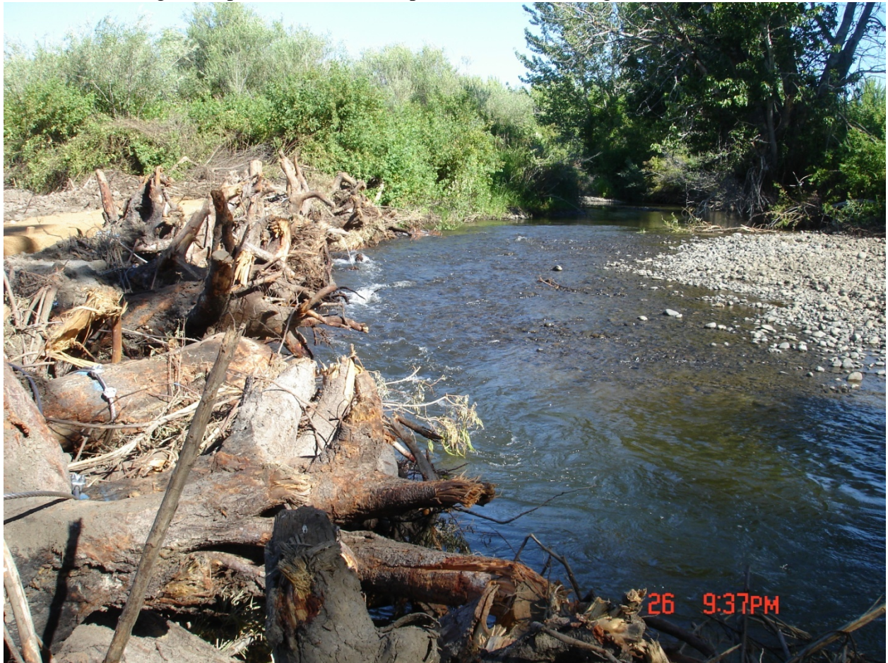
Figure 10. Where Ahtanum Creek used to access farming road during high flows. Bank stabilized to keep creek in original channel.
