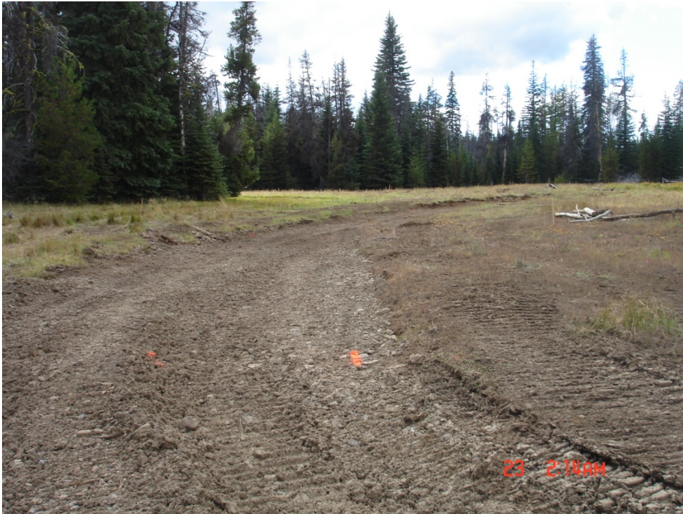
Figure 15. Lincoln meadows channel filled with compact soil and gravel.
