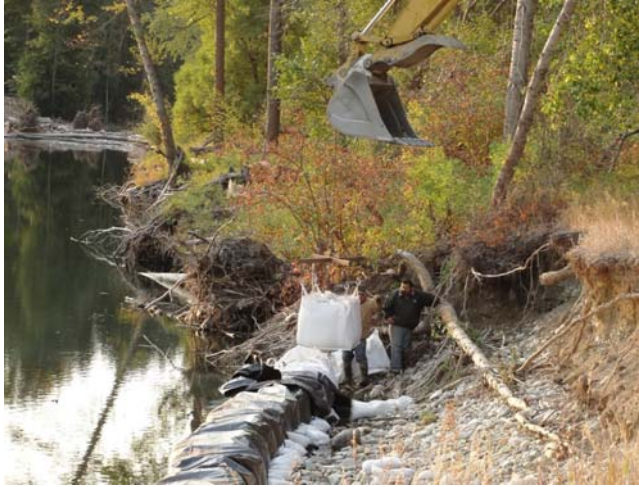
Coffer Dam Being Constructed
