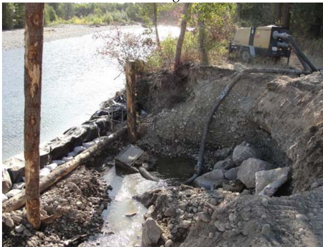
Sump For Pumping Water From The Coffered Area
