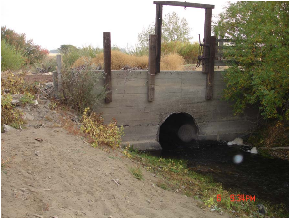
Figure 22. Graves culvert and headwall.
