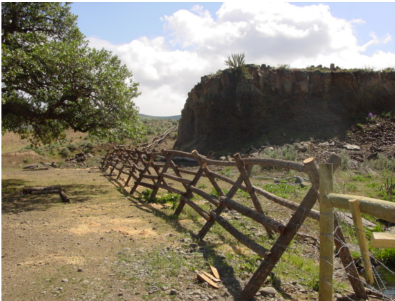
Figure 21. Buck and Pole Fence - Ahtanum Creek
