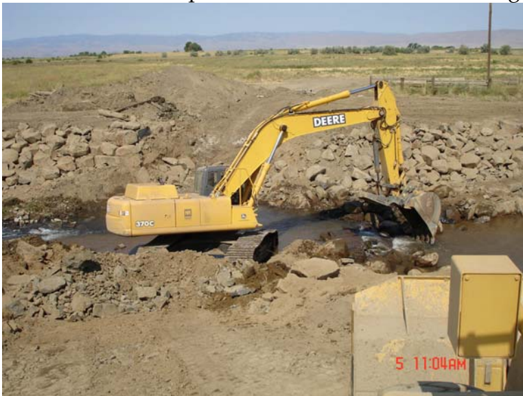
Figure 24. Excavator constructing grade controls.
