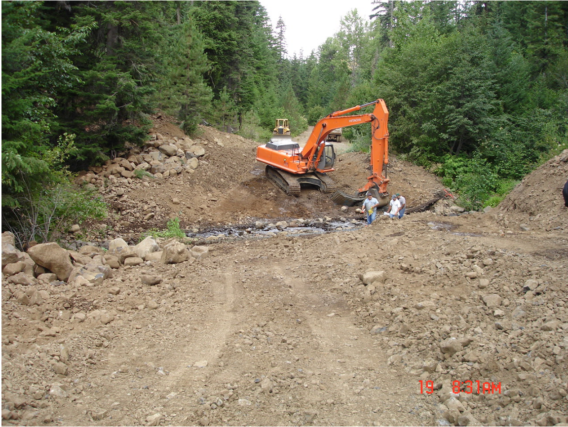
Figure 10. Construction of the new crossing approach
