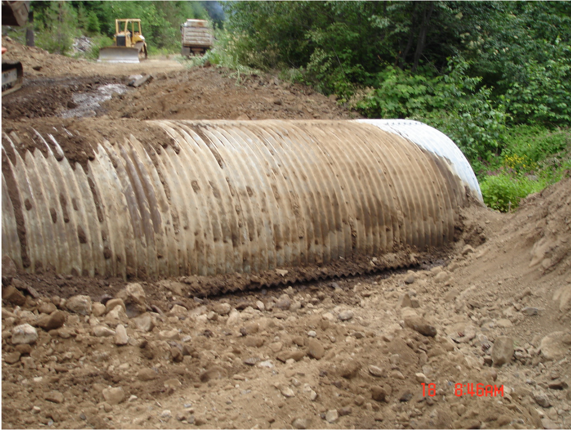
Figure 9. Lower culvert exposed by excavation
