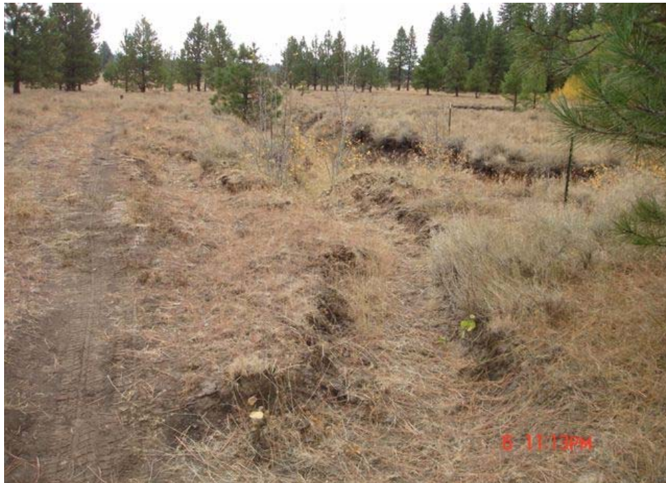
Figure 6. Road vectoring water into incised channel
