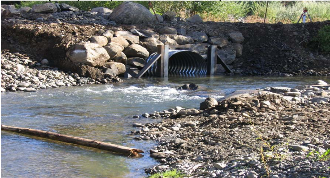
Figure 7 Ahtanum Side Channel Project Intake.
