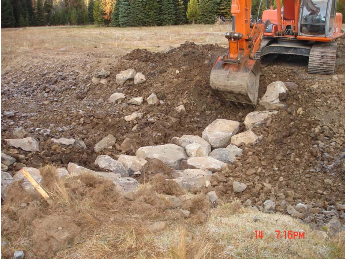
Figure 11. Grade control structure.
